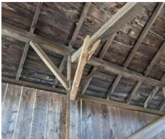
Village or Church Street Bridge
